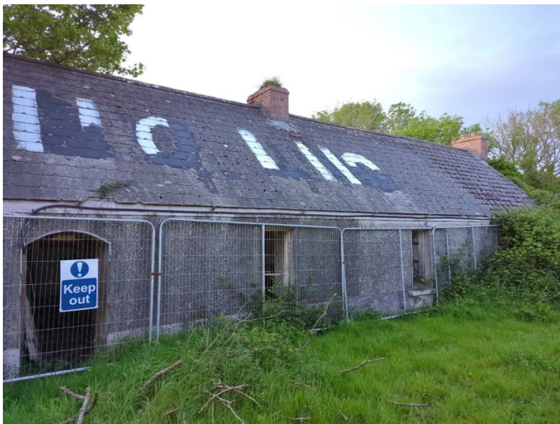
Photograph 18. Building 1 at location A located west of proposed development site
