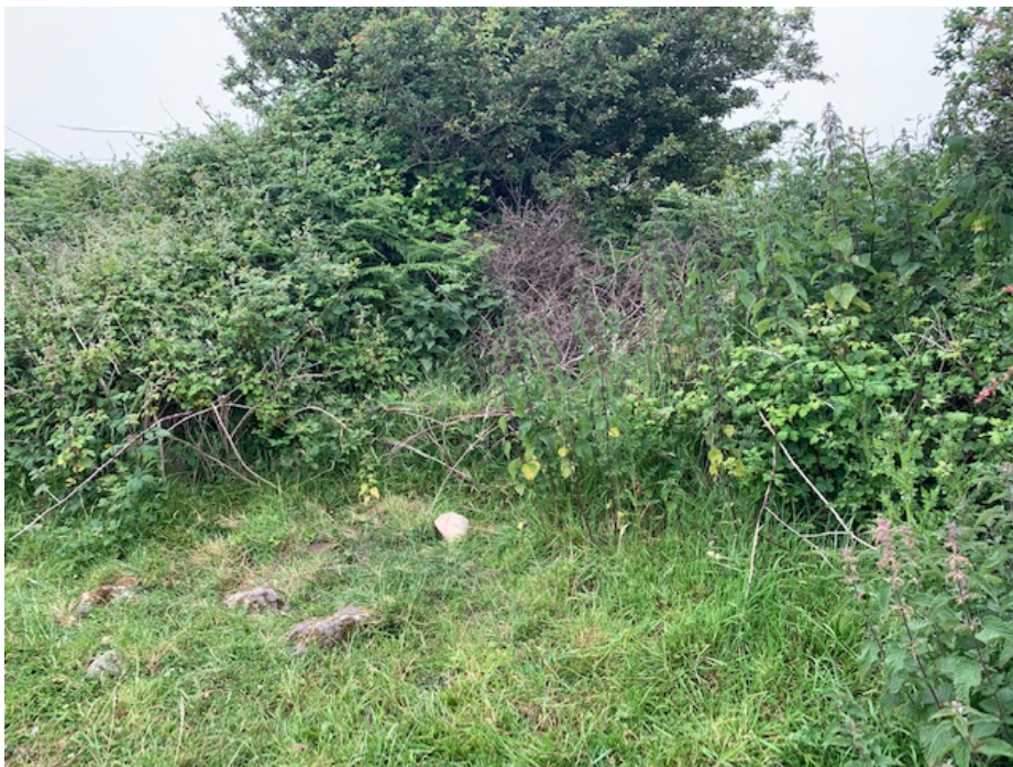
Photograph 12. Drainage ditch D4
