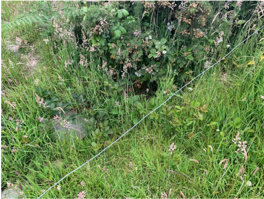
Photograph 11. Drainage ditch D3
