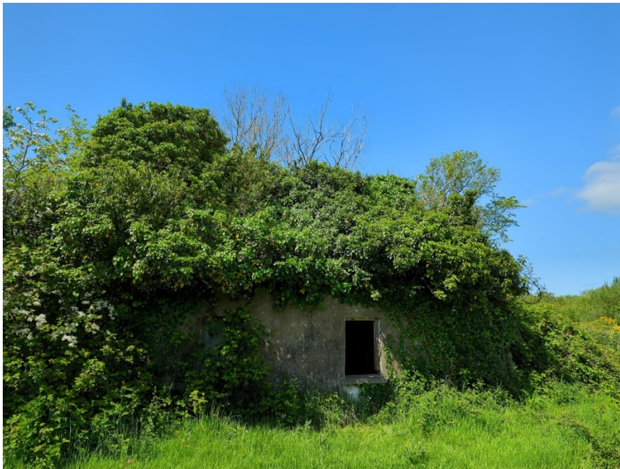
Photograph 16. Bat structure Location B within proposed development site
