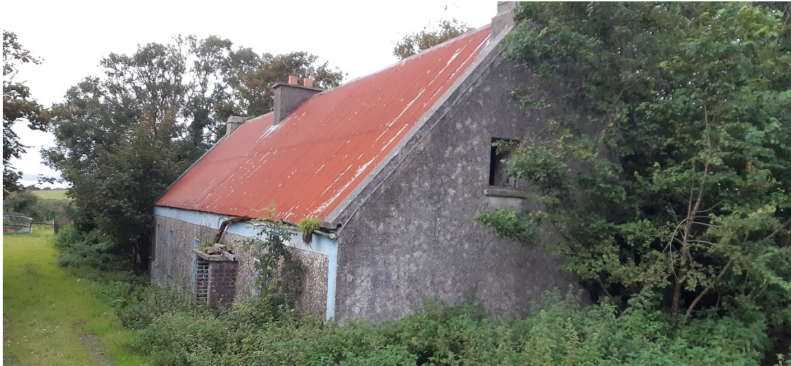
Photograph 19. Building 2 at location A located west of proposed development site
